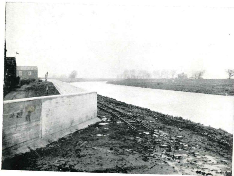
River Don. Ivy House. Retaining Wall completed.
