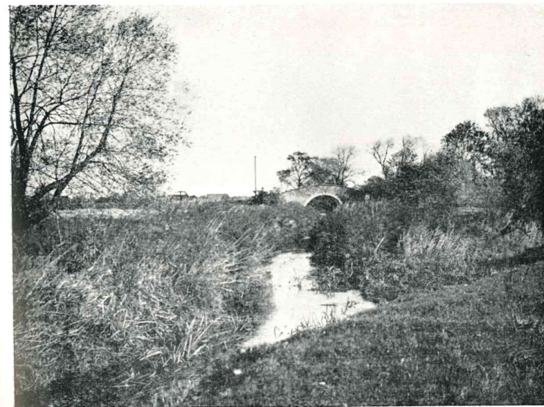
Foss Internal Drainage District. River Foss near Strensall before clearing.
