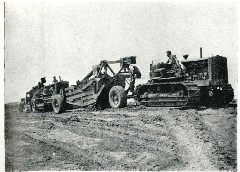
River Don. Tractors and Carry-All Scrapers.
