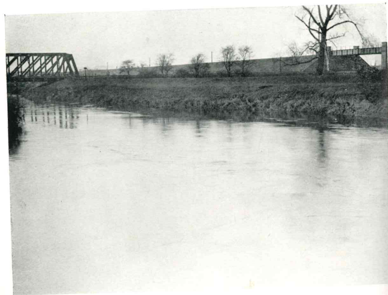
River Don. Weir removed.
