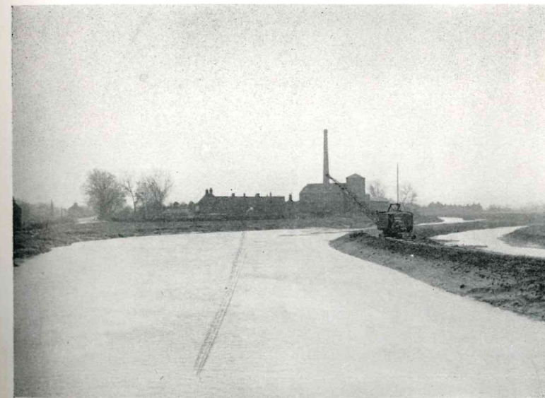
River Don above Jubilee Bridge. After improvement at bend.
