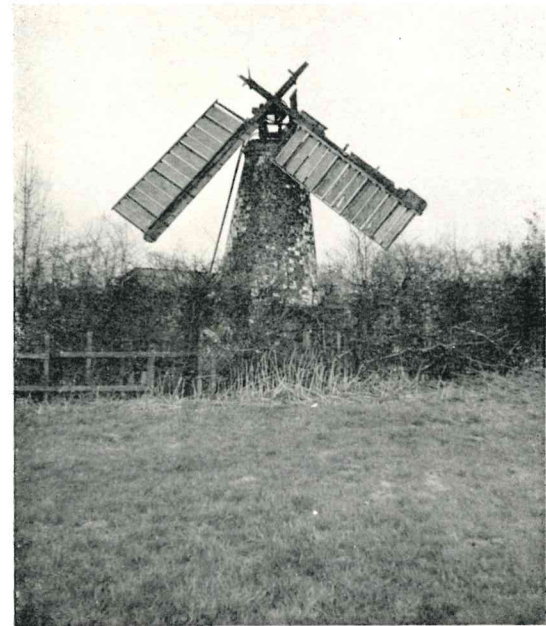
Acaster Internal Drainage District. Old Windpump.
