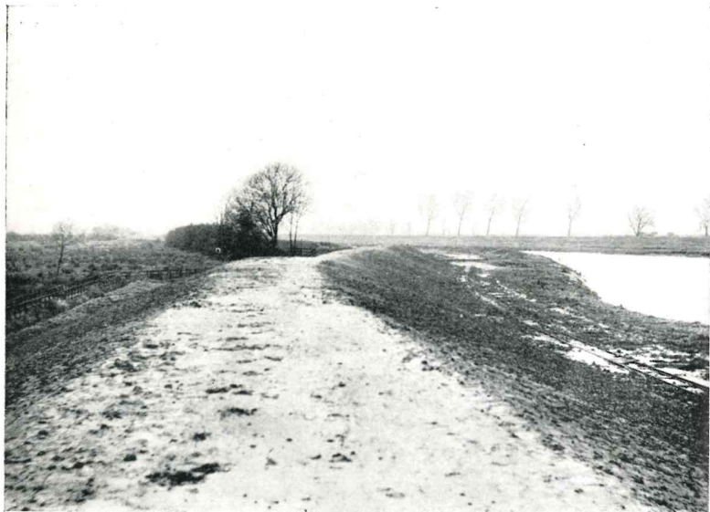
River Don. Embankment nearly completed.
