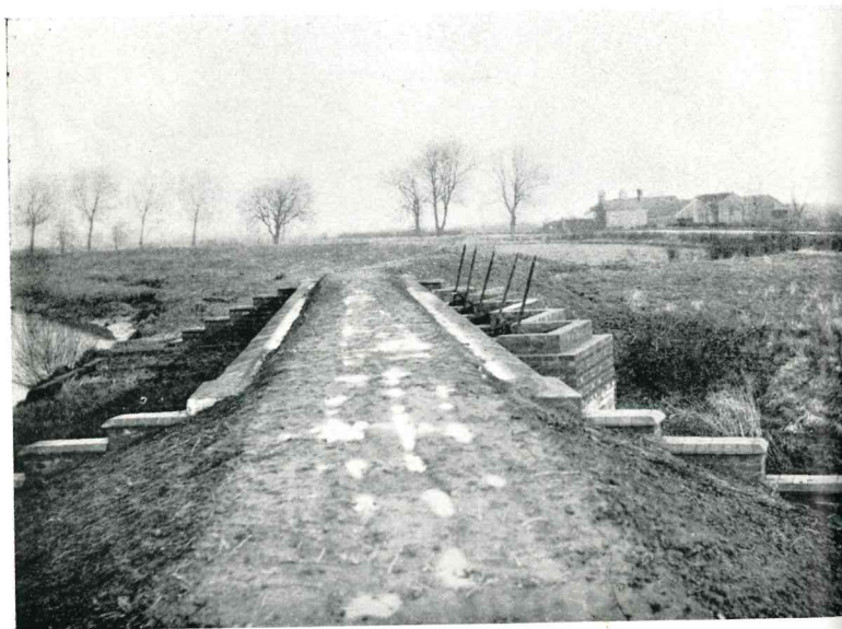
River Don. Durham's Warping Drain. Work completed.
