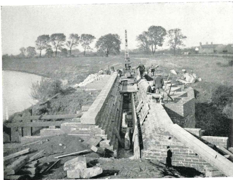
River Don. Durham's Warping Drain. During construction of walls.
