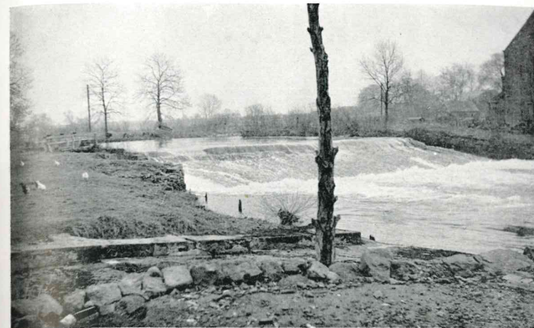
River Derwent. Elvington Weir. Before installation of automatic Sluice-gates.
