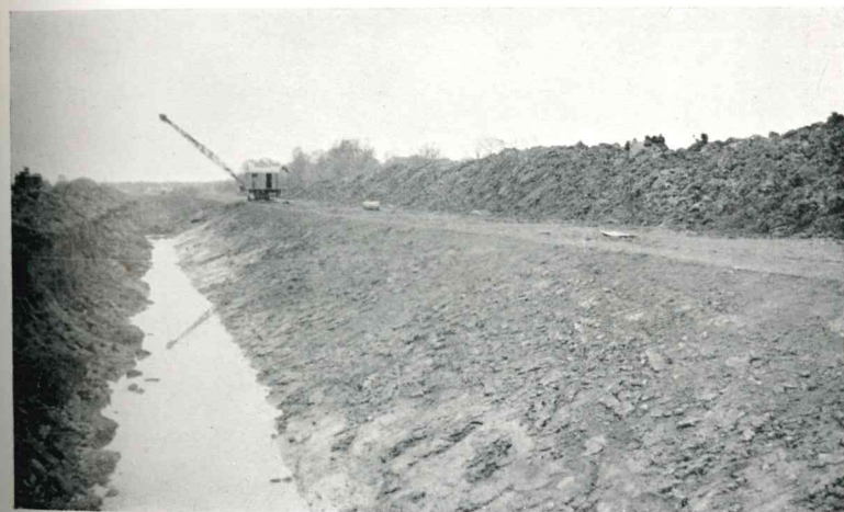
River Derwent. Sutton Diversion. Second operation.
