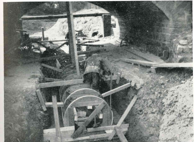
Dearne & Dove Internal Drainage District. Bulling Dyke. Forms for culvert shuttering.
