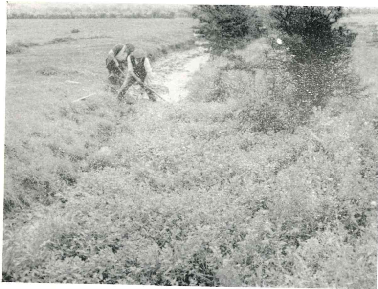
Dearne & Dove Internal Drainage District. Granewell Dyke before clearing.
