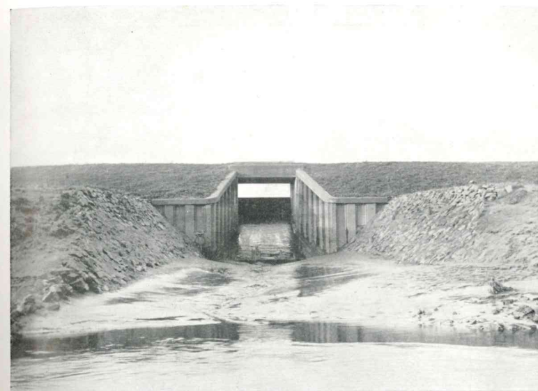
River Don. New Bridge. Canal Overflow and Ice Disposal Outlet.
