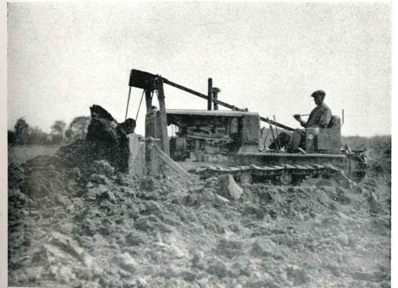
River Don. Bulldozer in operation.
