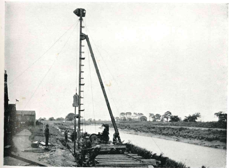
River Don. Ivy House. Pile-driver on site.
