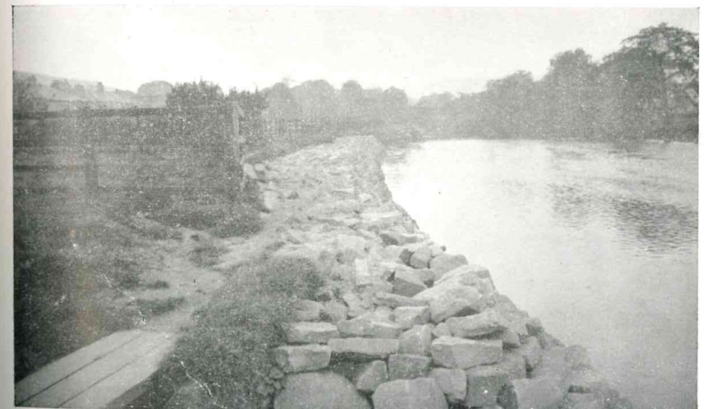
River Aire. Bingley. Rough stone wall to prevent erosion.
