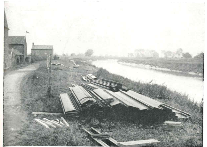
River Don. Ivy House. Site of Retaining Wall.
