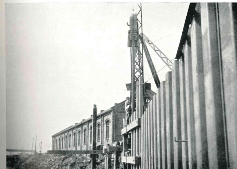
River Don. Rotherham. Illustrating height of Piling.
