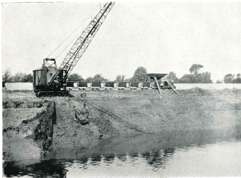
River Don. Widening and loading tip-wagons.
