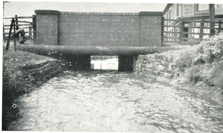
Dearne & Dove Internal Drainage District. North Dyke after clearing.
