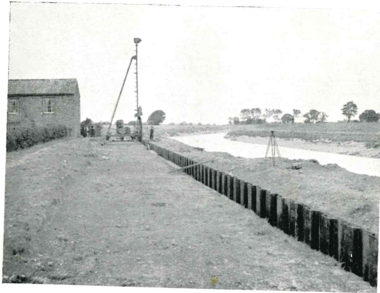
River Don. Ivy House. Sheet steel piling for Retaining Wall.
