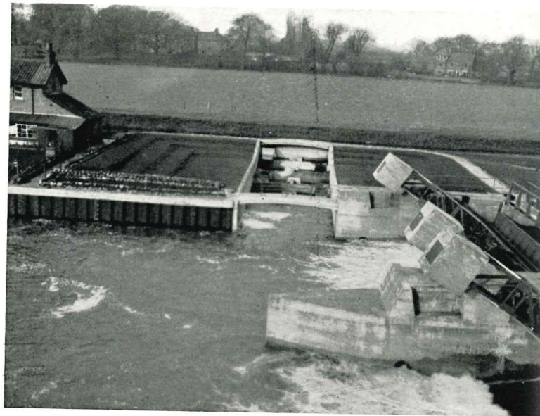
River Derwent—Elvington. Automatic Sluice Gates and Fish Pass.
