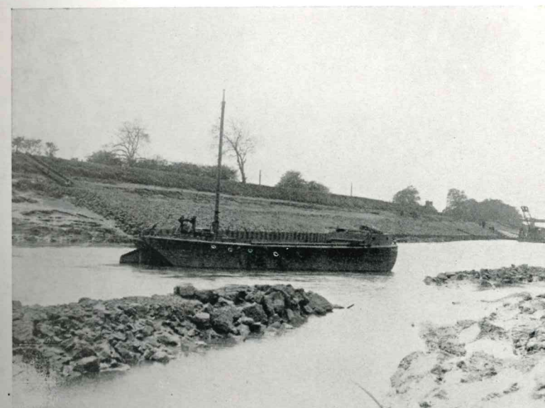
Stone deposited behind piling.
