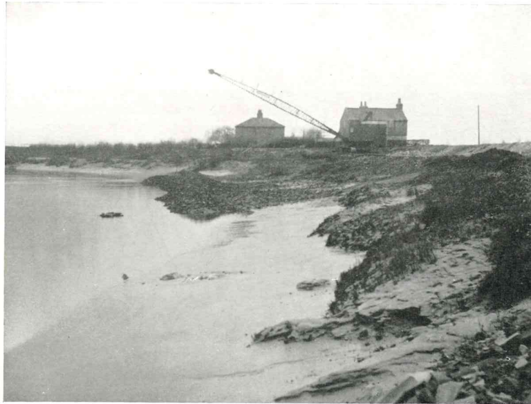
River Don. Stone deposited to form training wall at bend.
