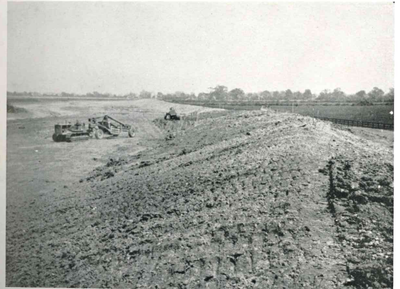
Forming new embankment. A further operation.
