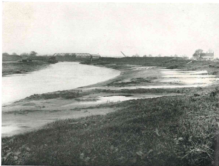
Deposited stone covered with warp.
