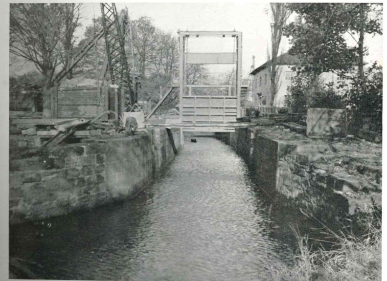
Sluice erected.
