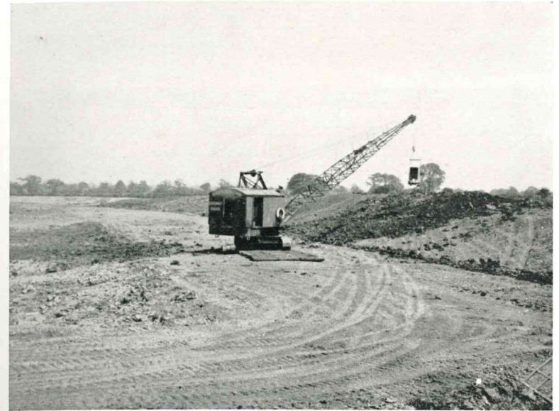
River Don. Forming new embankment.
