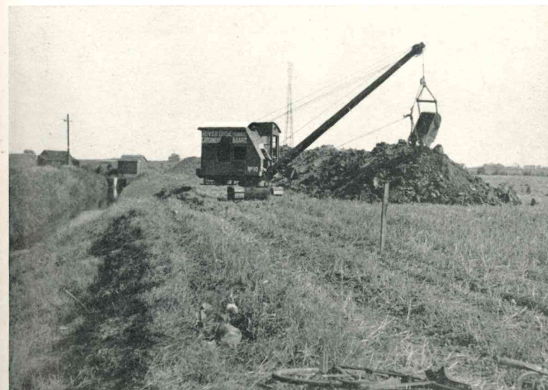
Snaith Internal Drainage District. Widening Main Drain.
