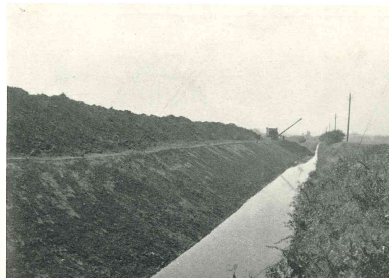
Snaith Internal Drainage District. Widening Main Drain.
