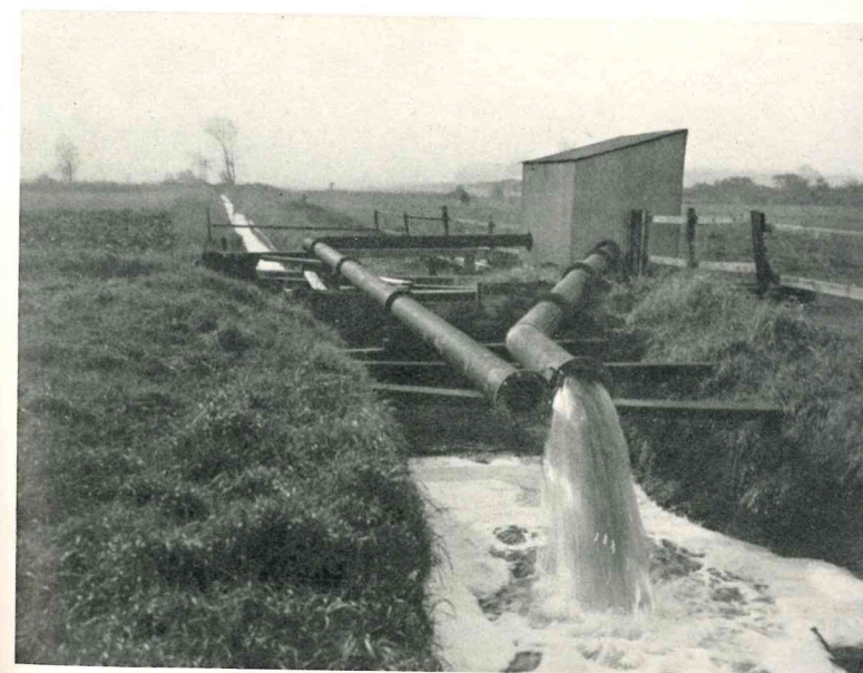
Colliery Remedial Drainage Works. Temporary pumping station, Great Common Drain, Askern.
