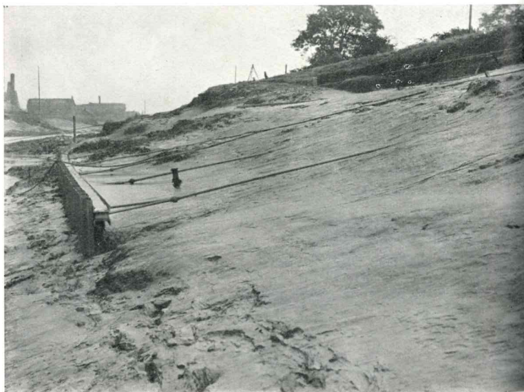
Dutch River. Tie-rods anchoring Steel Sheet Piling.
