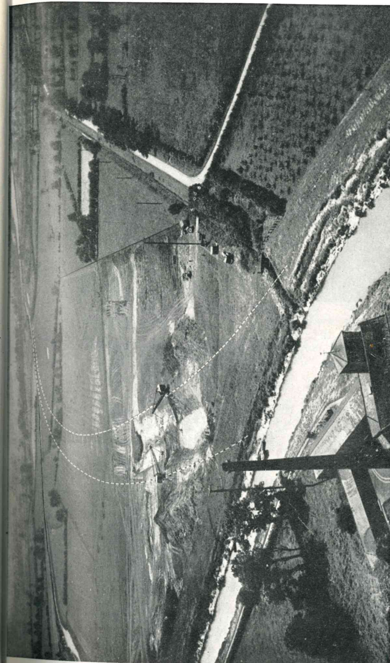
River Don. Commencement of diversion of Waterside, Thorne. (Line of diversion shown by dotted line). By courtesy of Priestman Bros., Ltd., Hull.
