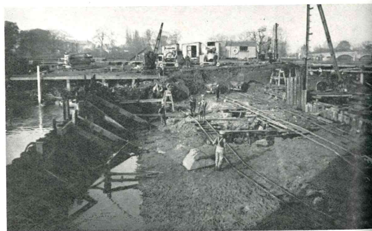
River Derwent. Elvington Weir after removal of crest.
