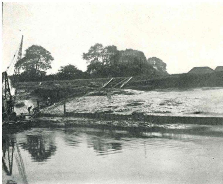
Dutch River. Typical length of Steel Sheet Piling.
