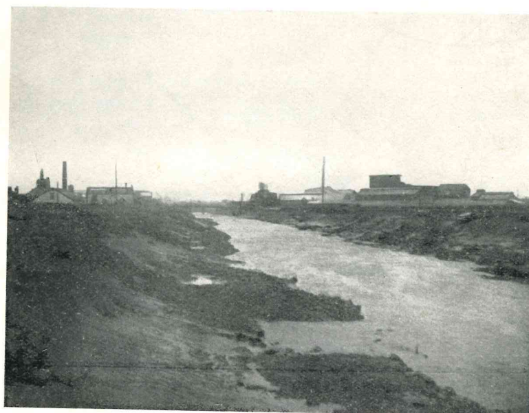
Dutch River. Shoal caused by slip in bank near Goole Railway Bridge.
