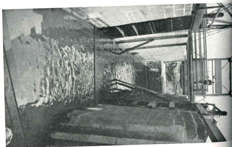
Elvington Lock. River Derwent. After construction of concrete floor.
