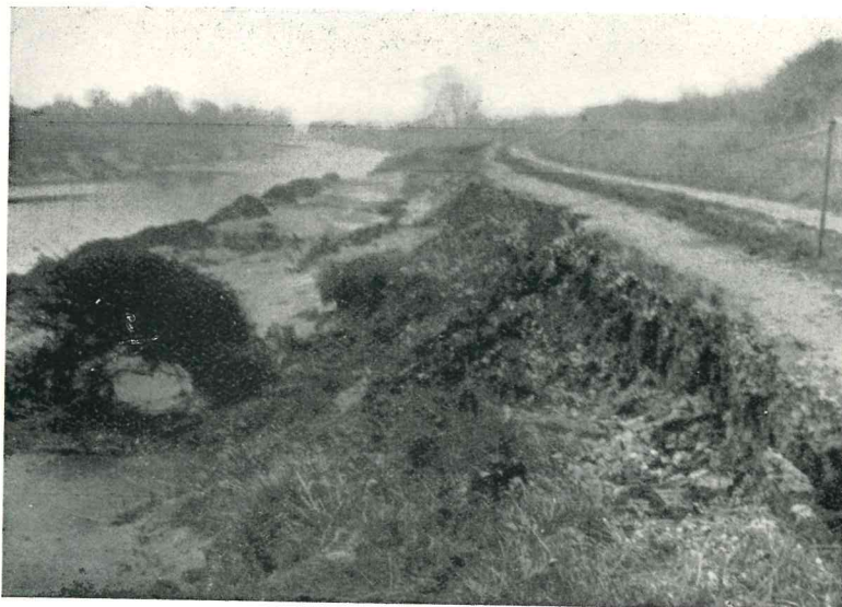
River Don. Typical slip in bank near Wormley Hill.
