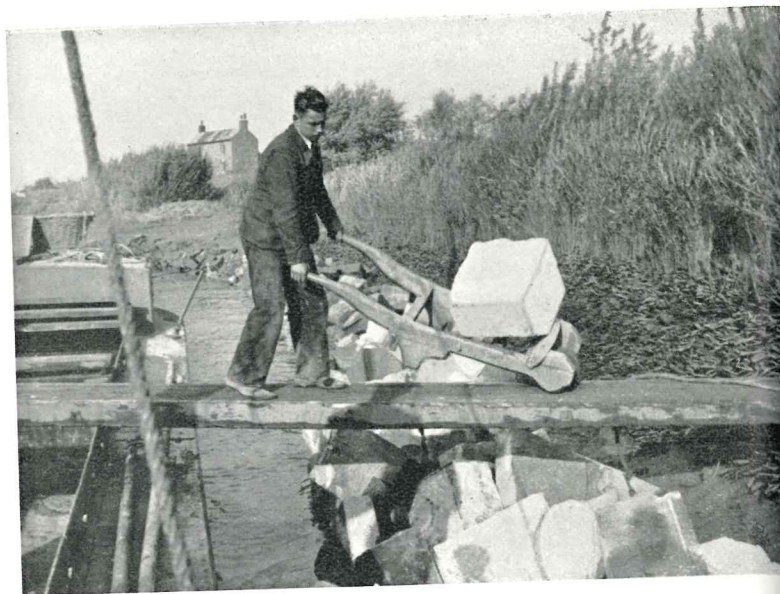
River Ouse. Wheel Hall bank. Depositing stone at toe.
